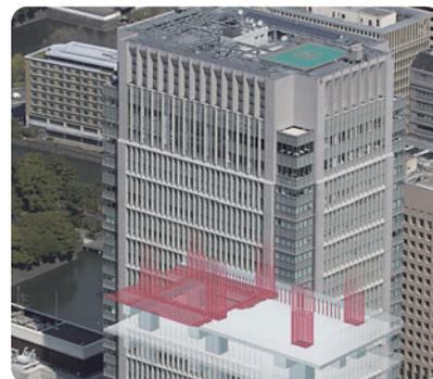
Tough Threaded Rebars are high-tensile threaded rebars used for structures built by connecting rebar, including high-rise buildings, roads and railroad support beams.
