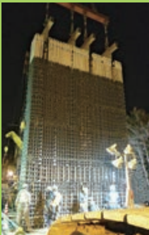
Positioning rebars for the portion of the seawall that extends beneath the surface into the bedrock to form the foundation of the structure. (Photo from the website of Chubu Electric Power Co., Inc.)
