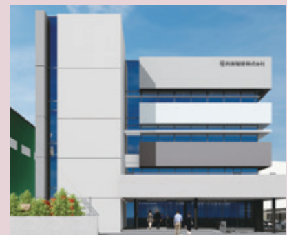
Yamaguchi Division: Illustration of completed new office
