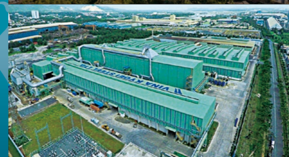
Vina Kyoiei Steel Co., Ltd. Ba Ria-Vung Tau Province, Vietnam (Established 1994)
