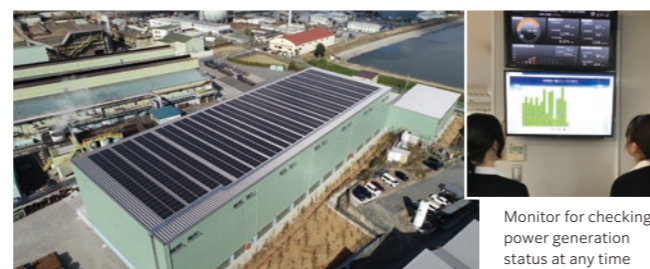
Product warehouse construction completed in July 2021
