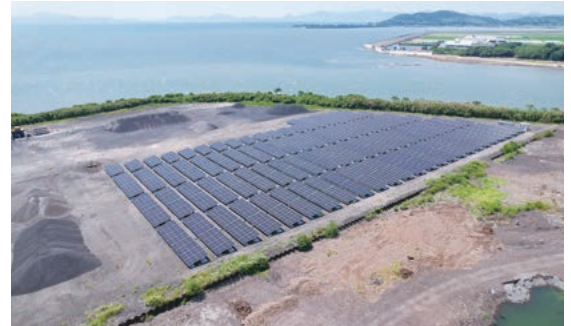
Higashioki solar power equipment
