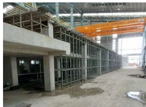
Foundation of the frame near the cooling floor
